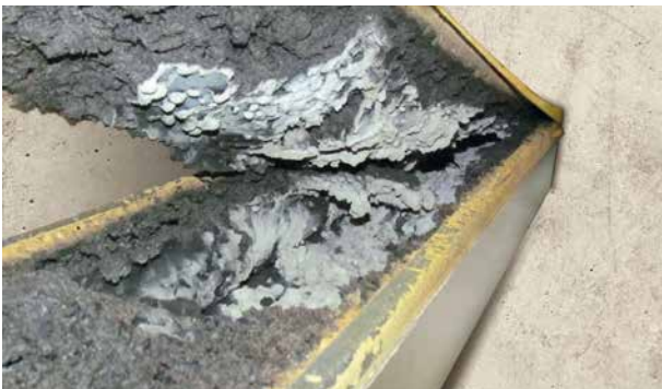
The foamed insulating material inside the cable duct prevents the fire from spreading
