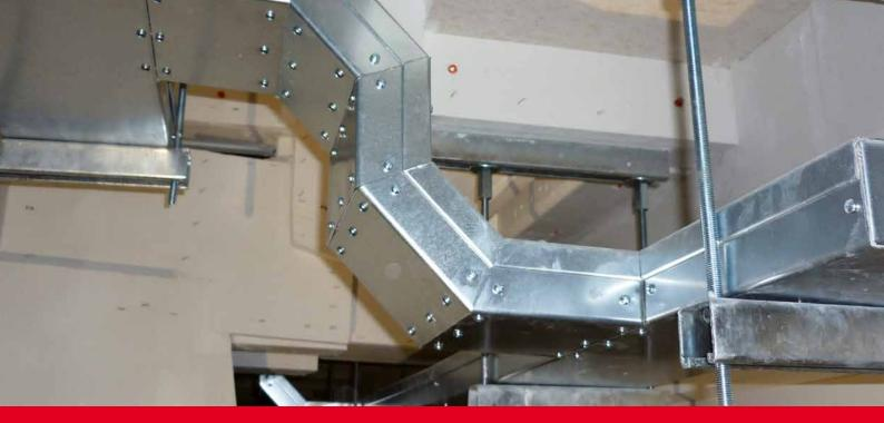
To ensure that the new ECB headquarters be equipped with state-of-theart fire protection technology, G+H Insulation was commissioned to install its innovative fire protection system PYROMENT®-IK90. From the outset, it was essential that the solution should occupy the minimum possible space. With a thickness of 1.6–3.0 mm and a weight of 6.5–10.5 kg/m<sup>2</sup>, the system can be installed even under challenging conditions. Moreover, the cable duct can be adjusted quickly
