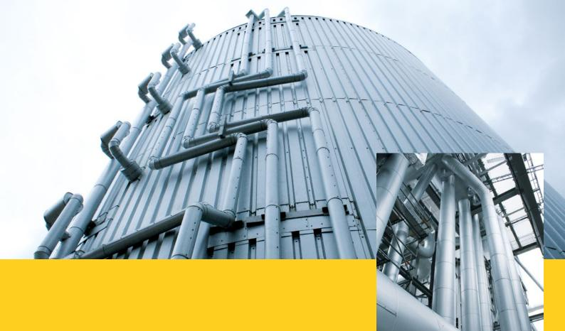
G+H Insulation technicians laid mineral wool mats with the RAL quality mark around the components to be insulated, which must withstand temperatures of up to 600 degrees. Afterwards, the installers completely covered them with aluminum-zinc sheeting. The metal components needed were customized on-site. Furthermore, G+H applied its fire prevention solutions to all steel structures in the refinery's fire hazard zones. To ensure that the bea-
