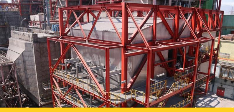
The heat and sound insulation was installed on ducts, E filters, fans, pipes and reactors. The insulation of the flue gas denitrification unit presented a particular challenge due to the high temperatures. In order to meet the European standards expected by the customer, G+H had shipped 95 % of the insulation material to Chile. In combination with selected materials, G+H Engineering were able to reduce the general problem of the thermal bridges. The insulation system also
