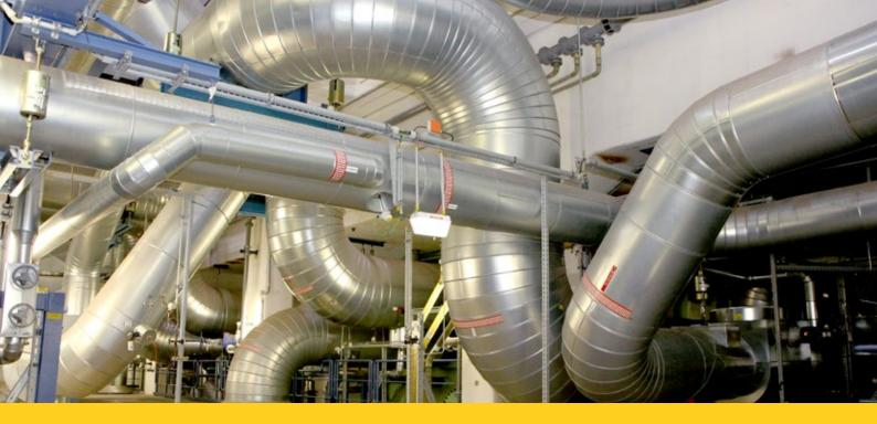
G+H installed thermal insulation and soundproofing on all the vessels in the boiler and power house as well as on the plant's outdoor pipes. The vertical high pressure pipes were up to 80 m tall and had to be insulated with multilayered materials containing special components such as CMS fibers. This was a challenge. Insulation materials are often mounted using double clamping rings. However, in this case, the extremely high temperatures and
