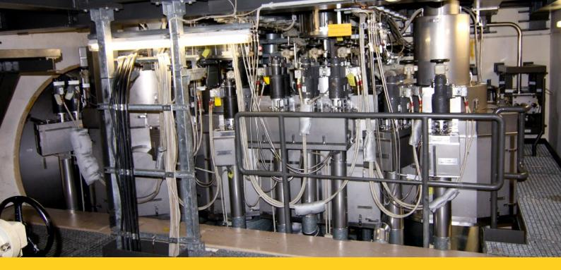
In the course of modernization of the Isar 2 nuclear power plant, G+H replaced the insulation of the SSV stations in the block. Using a 3D model that detailed all areas of the particular station, a custom-made insulation system was designed. This construction allows partial deinstallation and reinstallation of all insulation systems. In total, G+H mounted 80 ISOCAP® insulation cassettes and mattresses with thicknesses between 20 and 220 mm on each loop of
