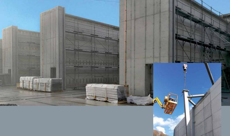
The transformers are housed in four cells, on whose walls the experts from G+H have installed the SONEX® W sound absorbing wall lining with an insulating thickness of 100 mm and a wall clearance of 50 mm. They have also fitted four acoustic doors to provide access. The cells are closed from the front with craneable stoplogs. These can be removed if necessary so as to permit access to the transformers when, for example, maintenance work
