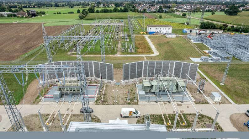
To improve noise control, two SONEX®-T screening walls from G+H Noise Control, with an overall length of 33 metres and a height of 8.5 metres, were installed at the transformer substation in Weier. The deployed screening wall elements are integrated into a special support structure, allowing them to be adapted to every local situation. This enables fast and easy assembly of the solid-wall elements. They are 120 mm thick and conform to a weighted sound reduction index (DW) of 47 dB.
