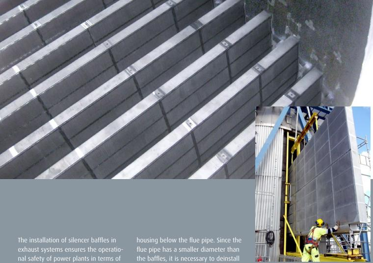
The installation of silencer baffles in exhaust systems ensures the operational safety of power plants in terms of noise control without hindering the flow of exhaust air out of the gas turbines. Replacing damaged baffles is essential not only to maintain noise protection, but also to preserve the mechanical protection. The baffles in the Halmstad power plant, which are up to seven by eight meters in size, are located in the silencer baffle
