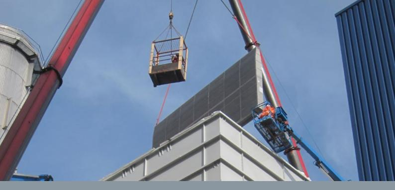
In order to prepare the Vilvoorde CCPP for its role as strategic reserve, the boiler was first taken out of operation. To do this, G+H installed a blanking plate up-flow of the boiler and a 45 m high bypass stack, which now provides the exhaust route for the flue gases. This system enables the power plant to start-up and cycle more rapidly. The silencer has several 10 x 10 m splitters and is integrated into the stack. This
