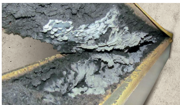
Foamed intumescent layer inside the cable duct prevents the spread of fire
