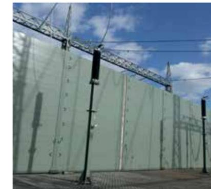
**Screening wall: a frame structure comprising I beams, sectional steels and edging to support the wall units**
