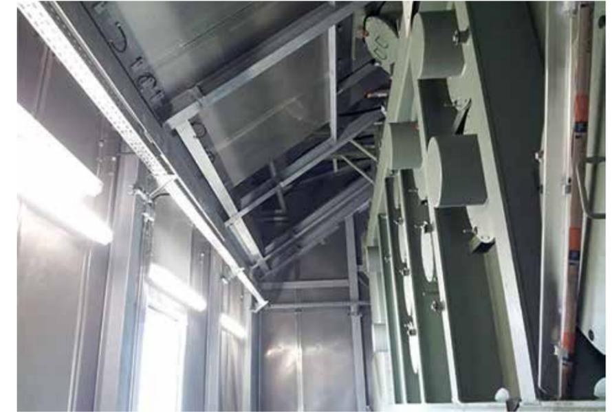
**Noise control housings (interior view): wall and roof elements rest on a frame structure comprising I beams and square tubes**
