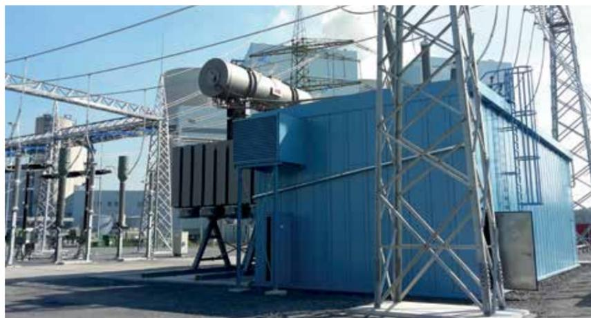
Transformer insulated with Sonex T including exhaust air silencer
