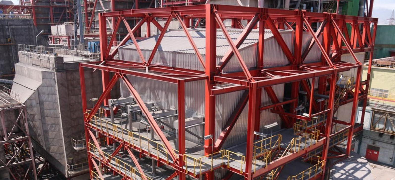
The heat and sound insulation was installed on ducts, E filters, fans, pipes and reactors. The insulation of the flue gas denitrification unit presented a particular challenge due to the high temperatures. In order to meet the European standards expected by the customer, G+H had shipped 95 % of the insulation material to Chile. In combination with selected materials, G+H Engineering were able to reduce the general problem of the thermal bridges. The insulation system also
