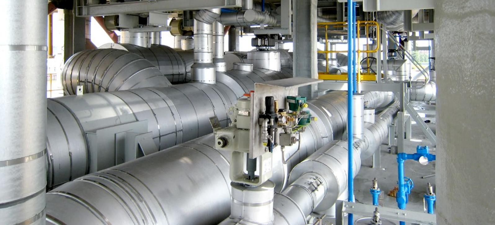
To organize the complex work processes as effectively as possible, G+H completely insulated the modules in a prefabrication hall owned by Hollandia in Krimpen (Netherlands). The customer transported the finished units by ship to their destination in England. Since there were a large number of pipes and equipment mounted next to and on top of each other on the modules, the low temperature insulation needed to be applied in a very tight space. To do this, a multi-layer cryoge-
